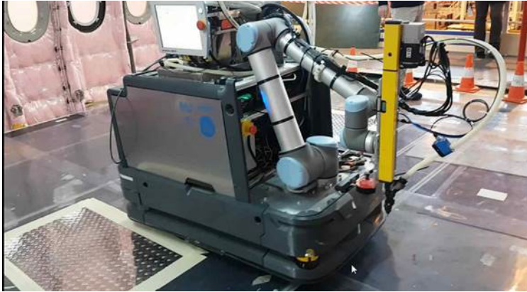
Floor panel installation
